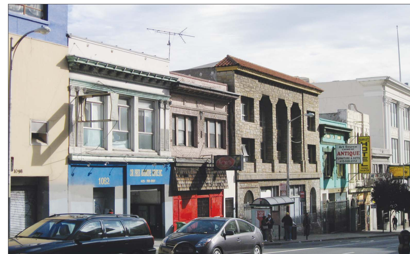
The seven buildings left to right on the north side of Geary all will be razed for the Cathedral Hill medical office building.
