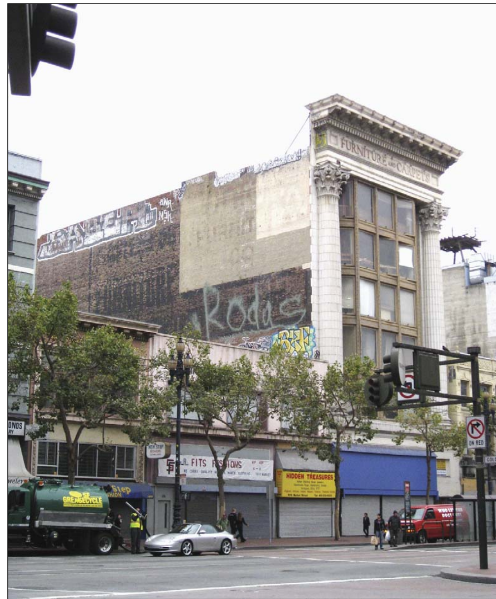
Furniture and Carpets , the store with Greek columns and classic facade at 1019-21 Market St., would be a candidate for one or more signs on the building's side if Proposition D passes.
