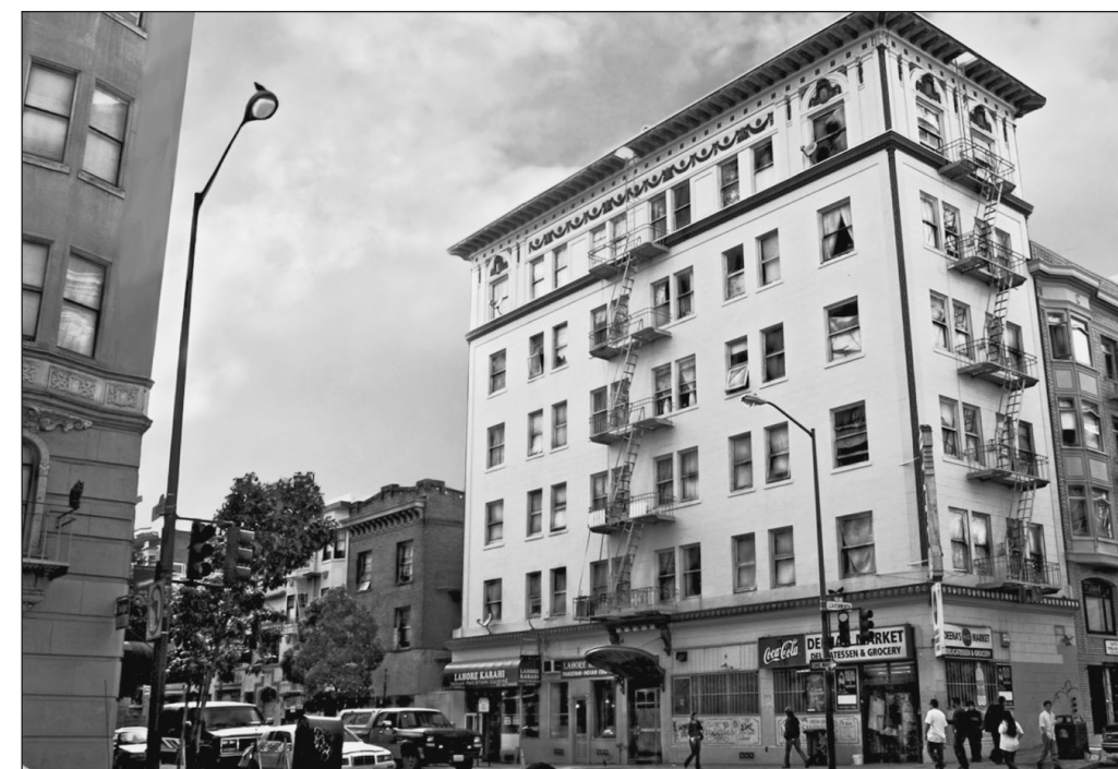
Under the wide projecting cornice of the Admiral Hotel, 608 O'Farrell, are garland reliefs, projecting cartouches above four of the windows, and a belt course that separates the top story.
