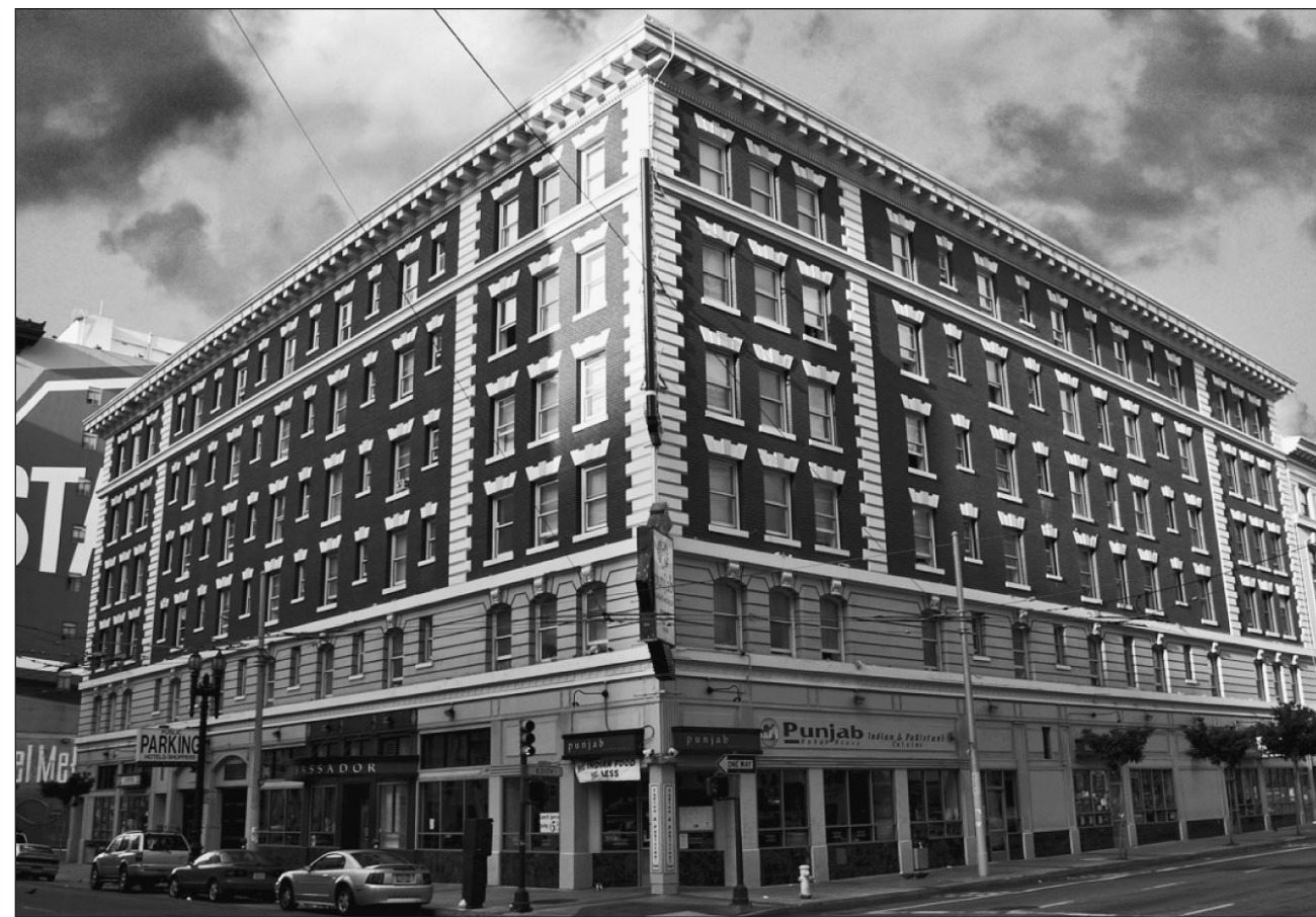
PHOTOS BY MARK ELLINGER TNDC's Ambassador Hotel, 55 Mason, built in 1922 by architects Earl B. Scott and K. McDonald, features quoining at the corner, ornamental lintels over windows, block moldings supporting the deeply projecting cornice, and horizontal belt courses, moldings that separate sections of the building.
