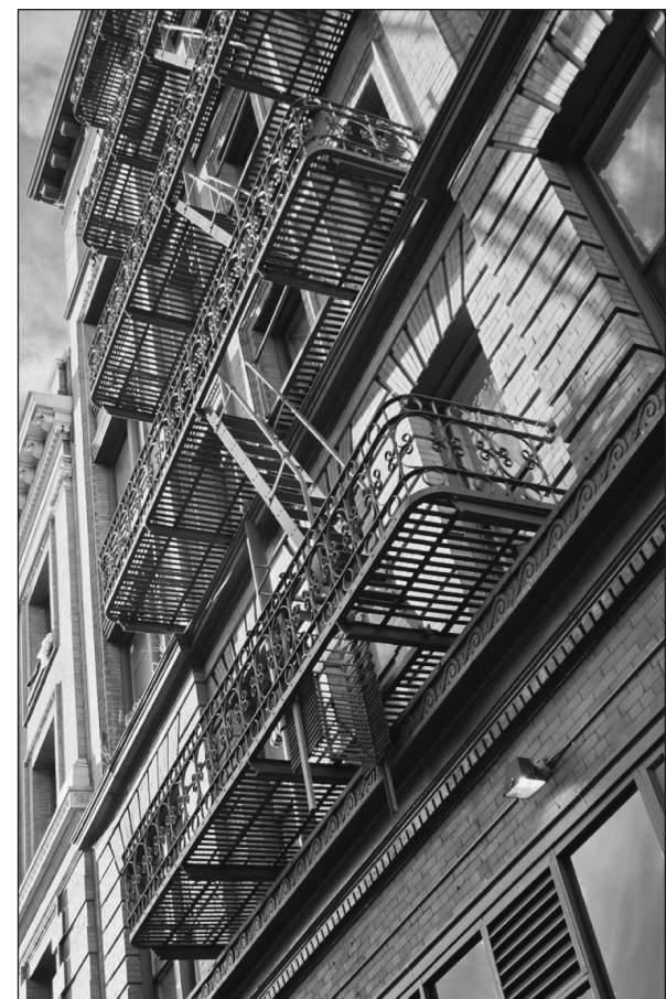
Incised brick around the windows, foliage on a projecting molding above dentils and decorative metal grillwork on the fire escape define the Empress Hotel, 144 Eddy.
