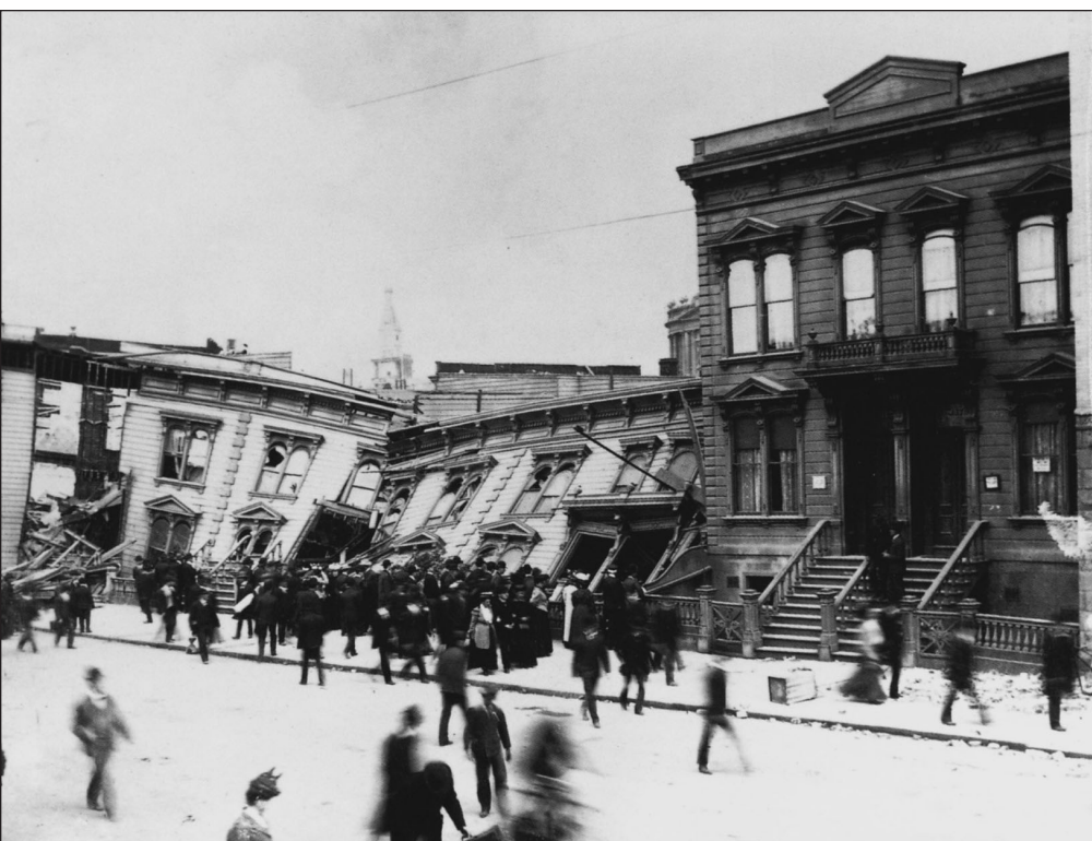
Golden Gate Avenue and Larkin Street after the quake, before the fire.
