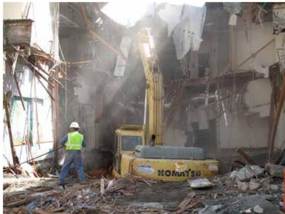
**A ghostly cloud** of dust rises from falling plaster and concrete, but a steady stream of water controls the air-borne particles.
