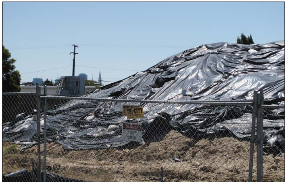
Contaminated soil on Avenue M is covered in black plastic to keep it from becoming airborne pending its removal.
